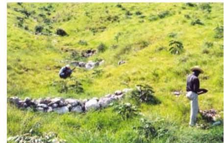
Gully plugs, Boucan Carre
